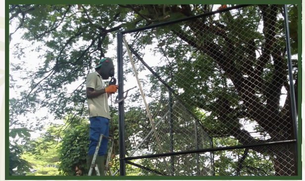
Construction worker, Leo, welding the strong mesh imported from Nigeria onto the frame.
