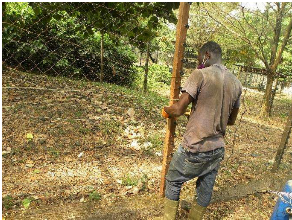
Installing new insulator poles in the mandrill enclosure
