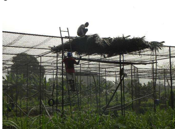
Replacing old palm leaves with new ones on the tantalus/patas enclosure
