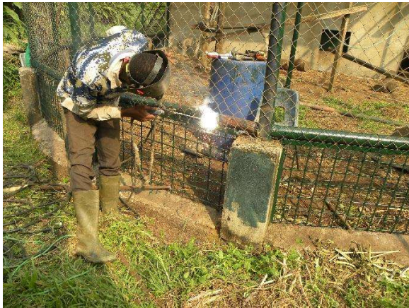
Cutting and repair of damaged structures in the red-capped mangabey enclosure
