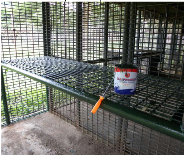
Repaired and replaced mesh are painted with a rust-resistant paint to increase their longevity
