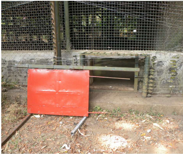
Old and rusted parts of the night dens had to be cut away and replaced
