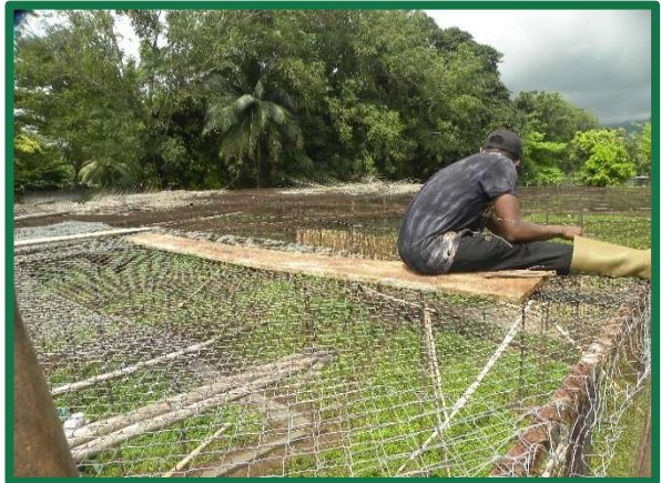
Repair of holes in the roof of the enclosure with new mesh
