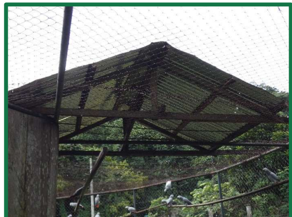
Permanent sun and rain shelters have been installed on the rehabilitation aviary to replace palm fronds and grass mats which rusted the roof mesh and encouraged snake activity.
