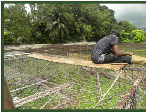
Making repairs to the roof.
