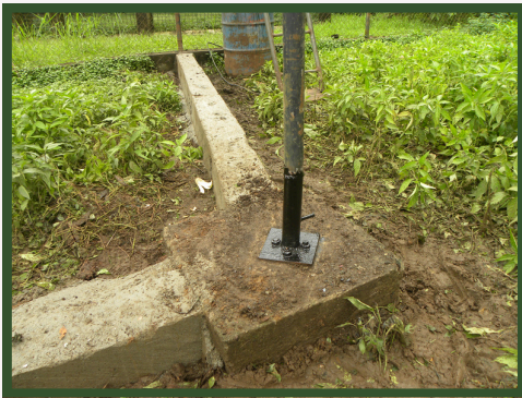
Building the partition inside.
