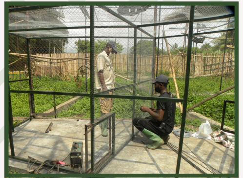
Building a new satellite cage.
